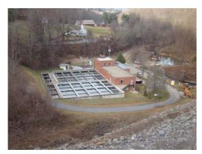
the capacity to produce 8 million gallons of finished water daily is producing slightly less than half that on the average, and it is backed by a reservoir and watershed which could supply 12 million gallons of water to the plant each day.
